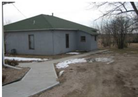
Ranch School Building (over 100 years old)
